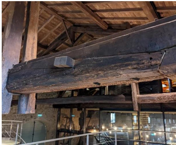
Figure 23: "Trait de Jupiter" joint at historic wood truss
