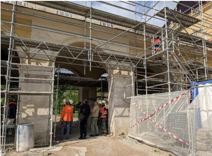
Figure 26: restoration of stone gallery
