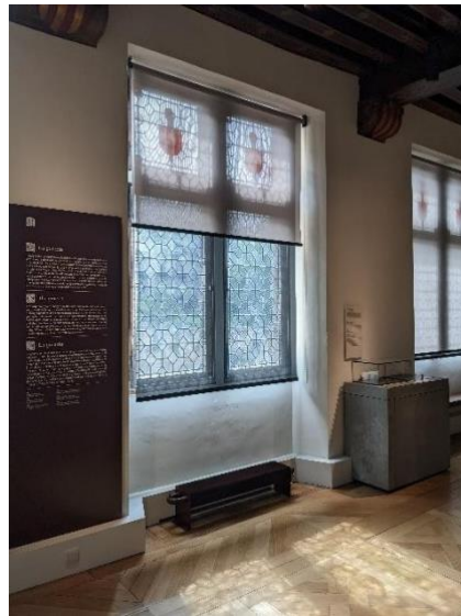
Figure 35: control of light levels at historic windows via multiple shades and films on glazing.
