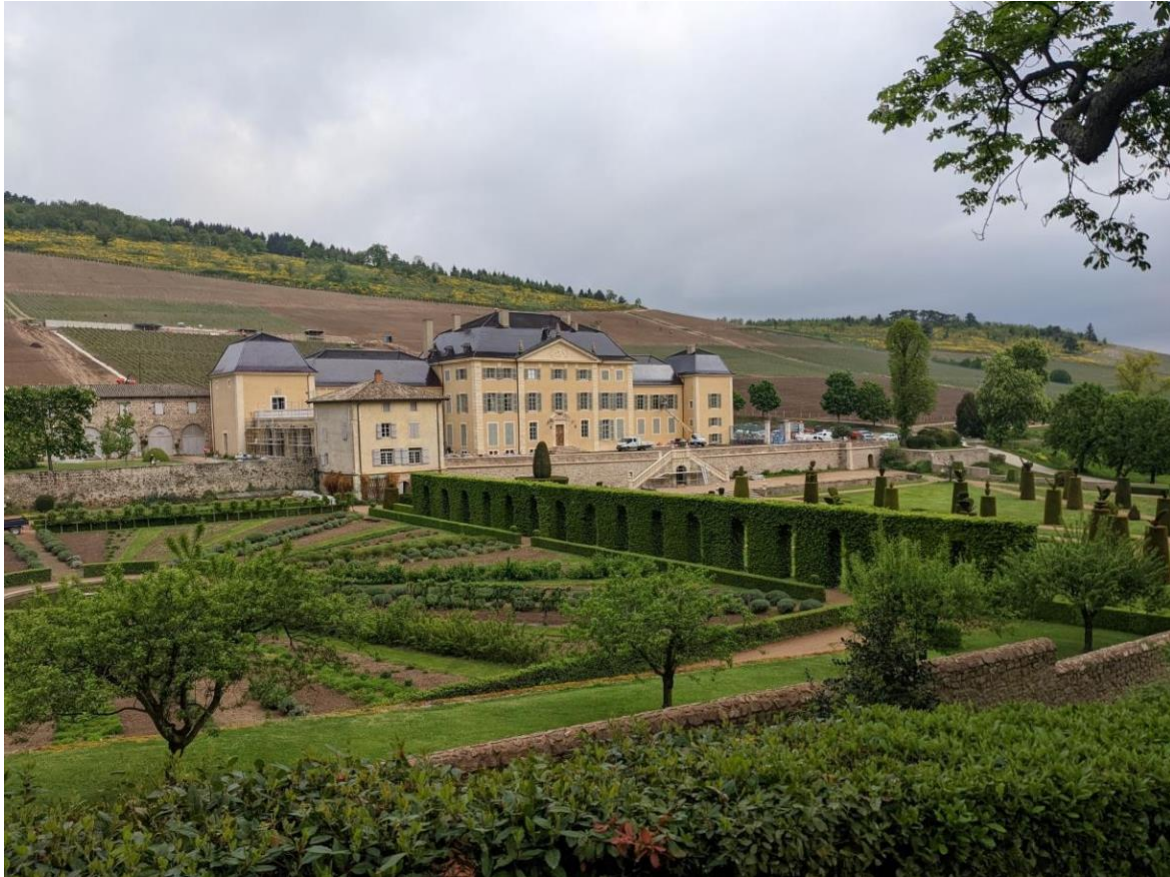
Figure 19: chateau with formal gardens at front and newly created vineyards on hill behind. New roof tiles recently installed.
