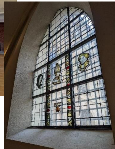
Figure 47, modern glazing layer added to protect historic windows.
