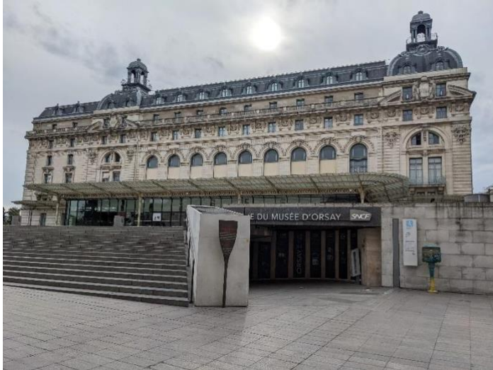
Figure 69: metro station below historic train depot.
