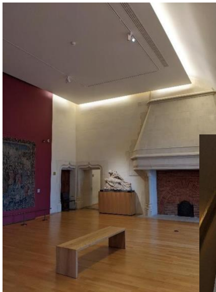
Figure 49, large volumes defined by planes of modern finishes hiding utilities.
