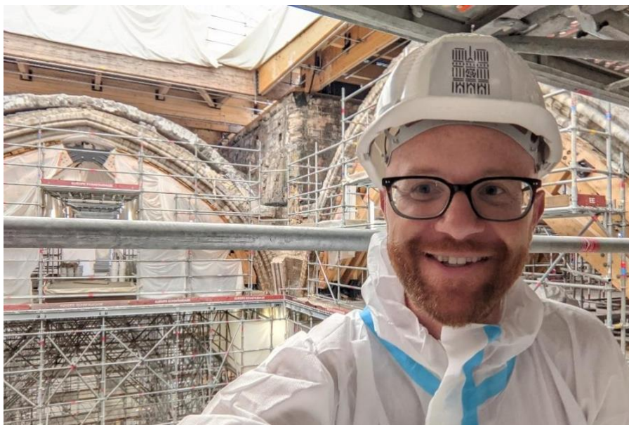
Figure 5: The author on a construction tour of Notre-Dame Cathedral. Full-body suits and decontamination showers were required as lead-mitigation strategies.
