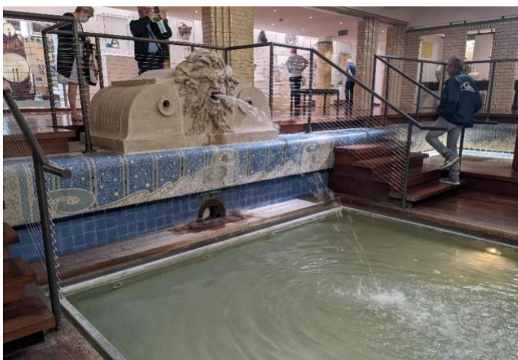
Figure 65: active water fountain at platforms within historic pool structure.
