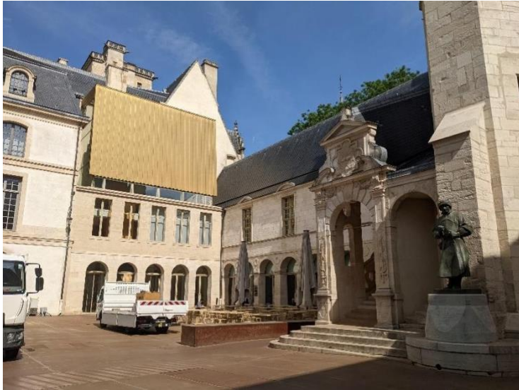
Figure 45, modern addition encloses stairs, mass is reduced with Mansard "roof," nested between historic structure.
