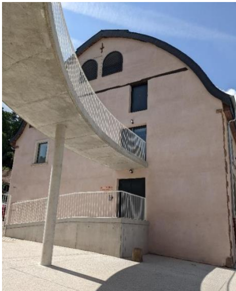
Figure 57: concrete bridge connecting museum to workshops.
