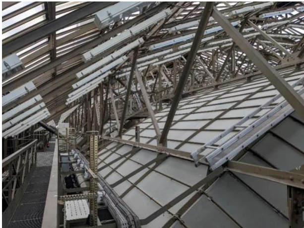
Figure 70: space between historic skylights and laylights.
