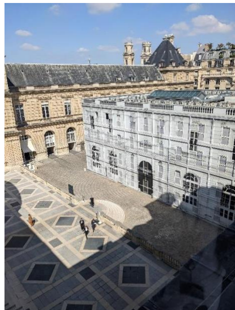
Figure 3: Portables that are beautifully integrated into interior courtyard, used as swing space so renovations can be phased over time, at the Senate/Palais de Luxembourg.
