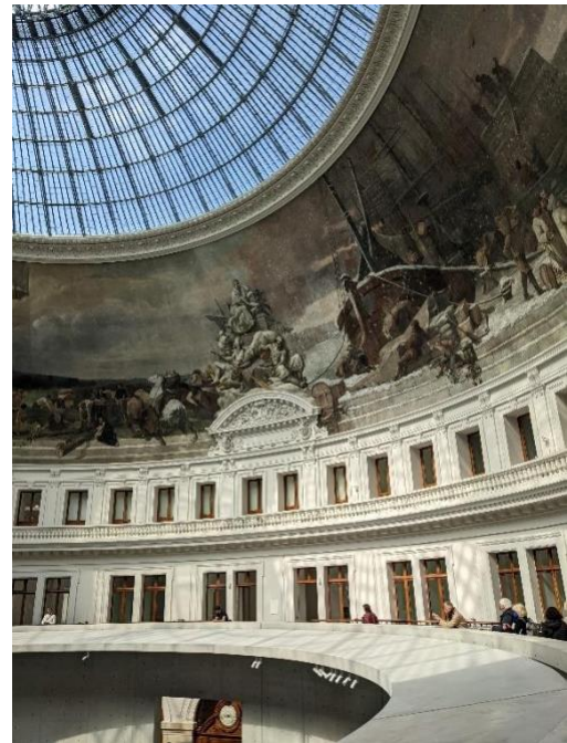
Figure 40, restored glass dome and murals, seen from top of interior addition.
