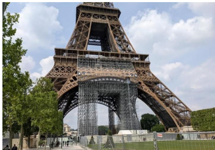
Figure 9: self-supporting scaffolding with decorative cover
