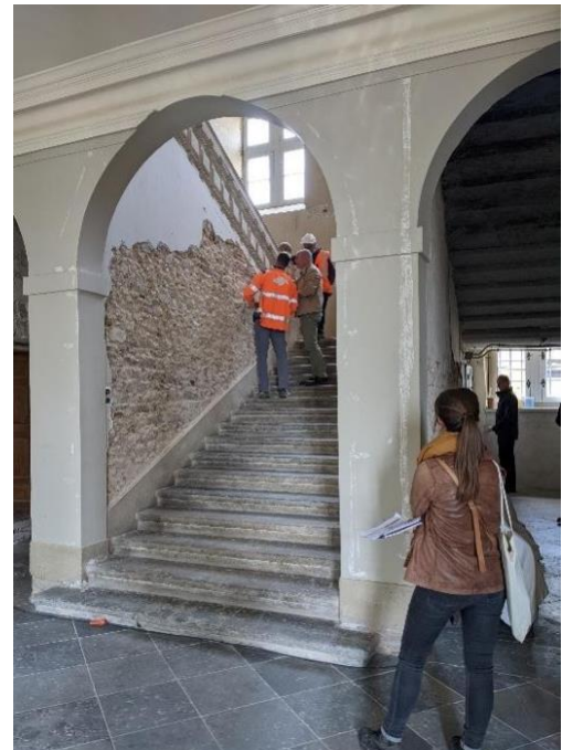
Figure 27: restoration of stone and plaster at interior
