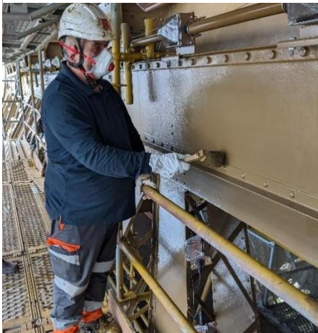
Figure 10: demonstration of historic brush paint application
