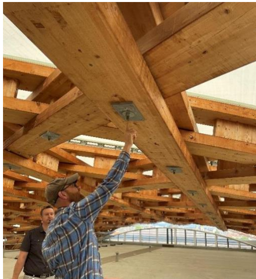
Figure 75: guided survey of cross-laminated lattice wood roof structure at Musée Pompidou-Metz.
