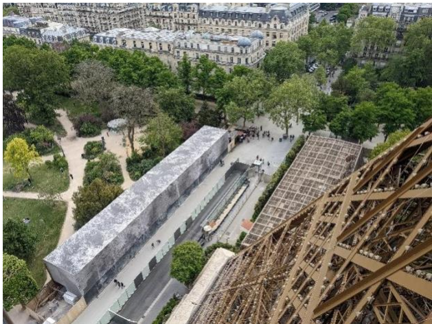
Figure 12: contractor work area hidden by decorative screens
