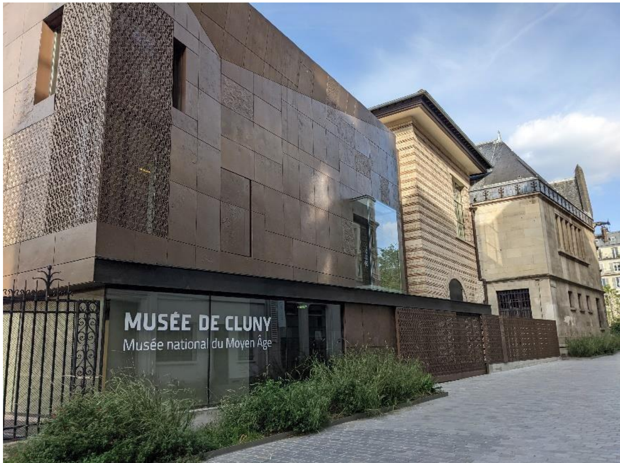
Figure 31: three different structures along urban path.
