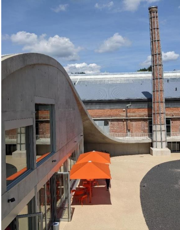
Figure 53: modern welcome center with undulating concrete roof/floor, connecting different structures.
