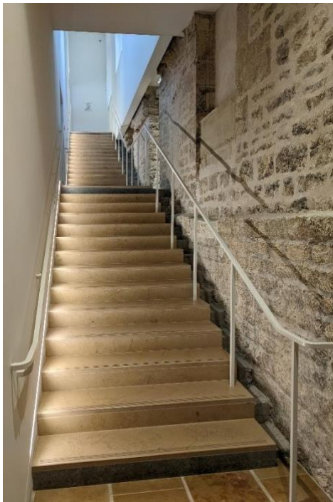
Figure 48: hollow joint to further visually separate new and old.
