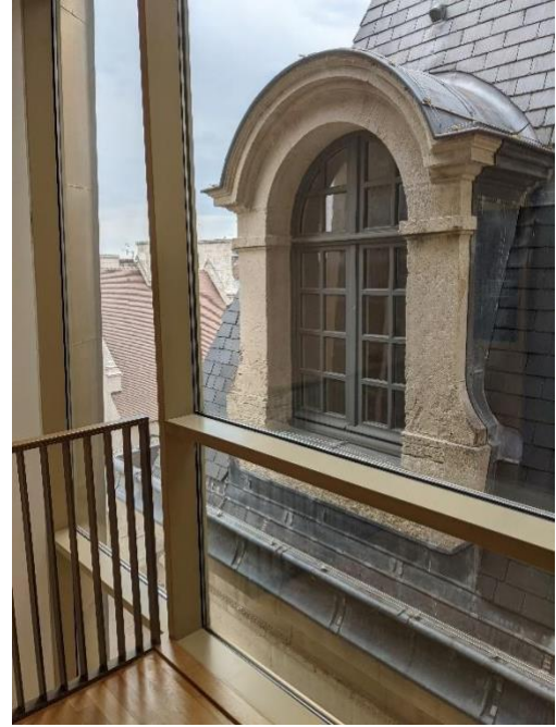
Figure 44: spacing between new and old at roof levels.
