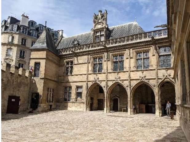
Figure 30: enclosed courtyard at abbey.
