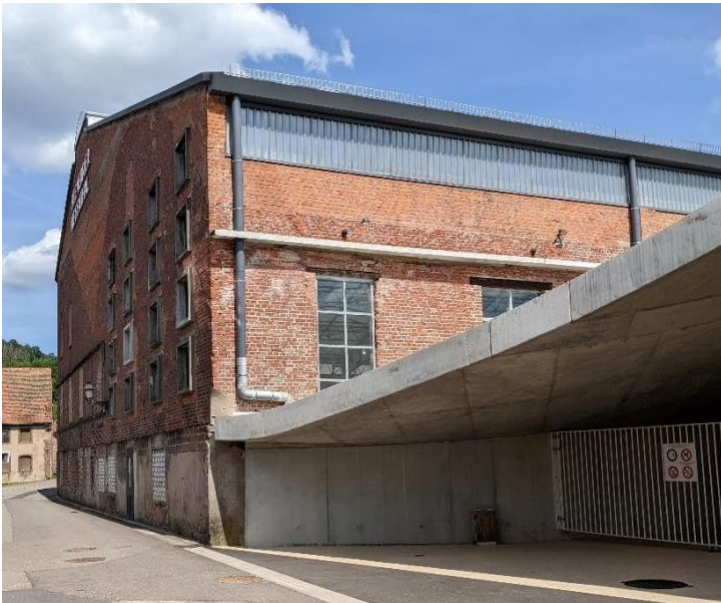
Figure 55: connection between welcome center and performance hall.
