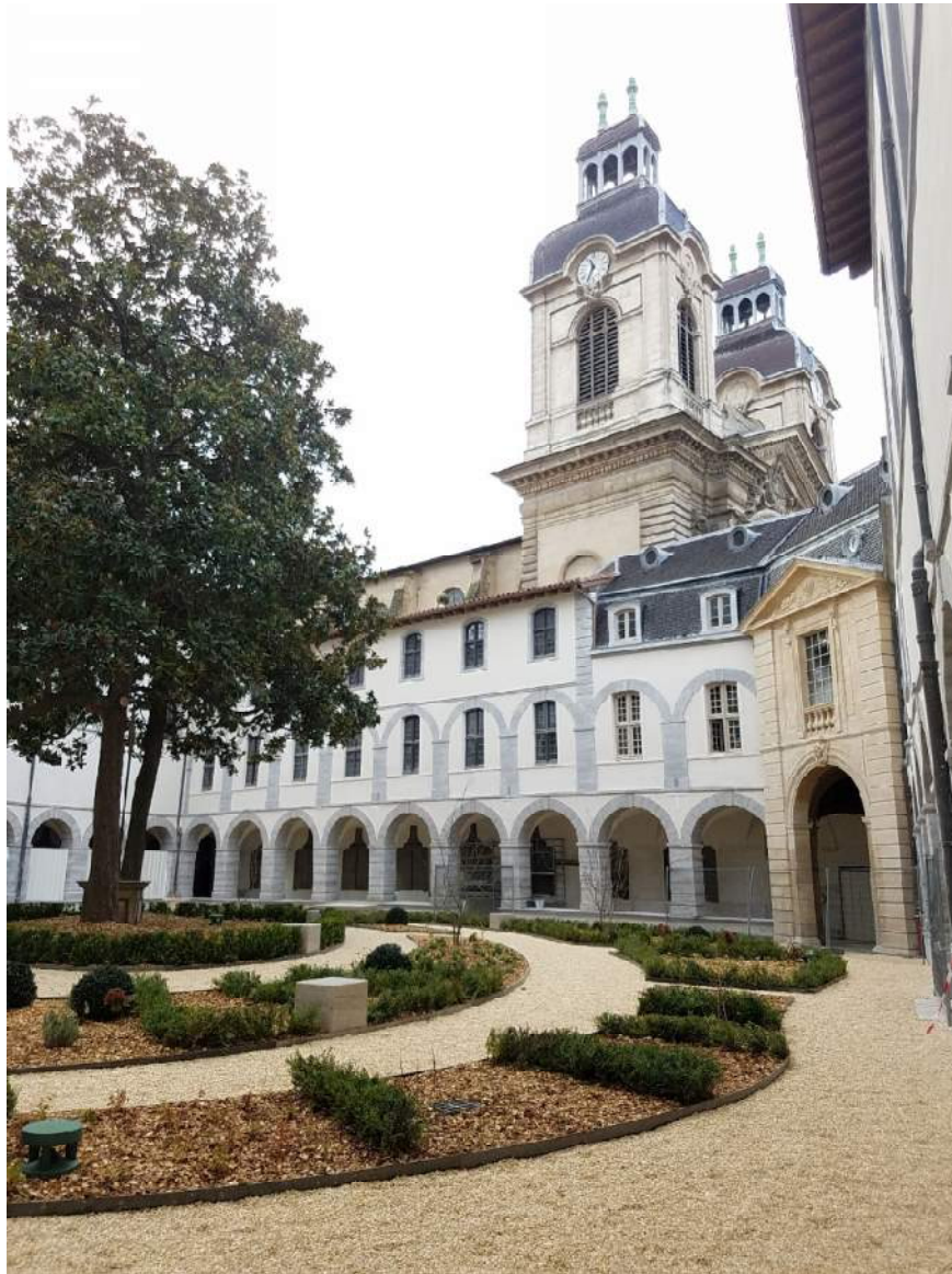
Fig. 5.1 Hôtel-Dieu de Lyon The restored cloisters of the old hospital (currently being converted into a hotel-conference facility). Constance Lai, December 9, 2018. Taken during a site tour led by Didier Repellin.
