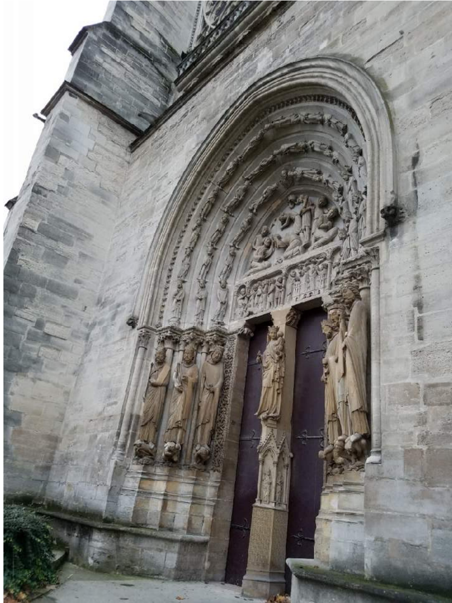
Fig. 7.4 North transept of Saint Denis. portail des Valois. The carved figures have darkened over time after the laser cleaning process was performed Constance Lai. December 1, 2017.
