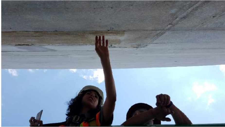
Fig. 7.1 NPS Conservator (government staff) and Masonry Craftsman (private company) reviewing the cleaning of marble stone with dry ice. Constance Lai. August 14, 2018.
